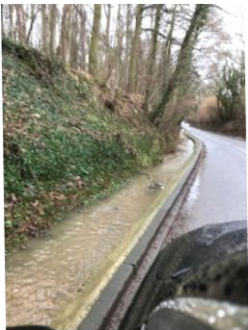
Image taken of Brickendon Brook after the renovation
